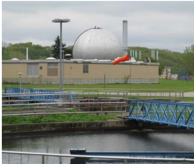
The Flint waste water plant that will be converted to produce biogas
